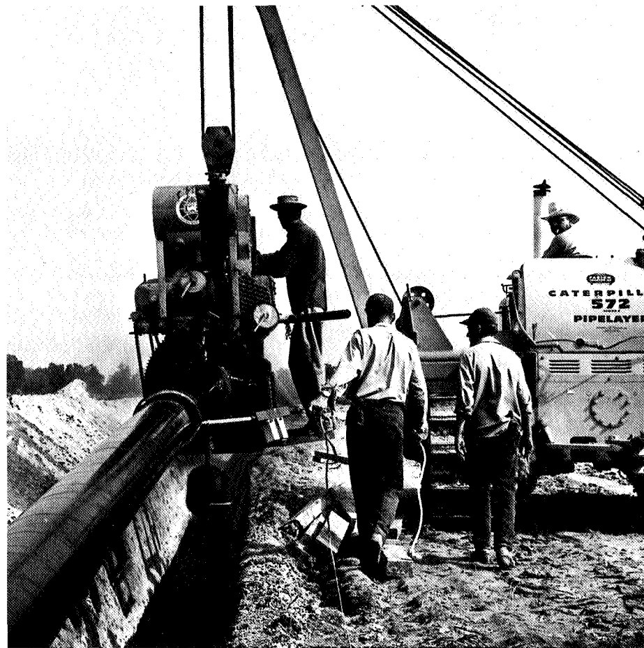
Pipeline construction specifications call for 36 in. of cover, but allow for 48 in. where deep plowing methods are used.
